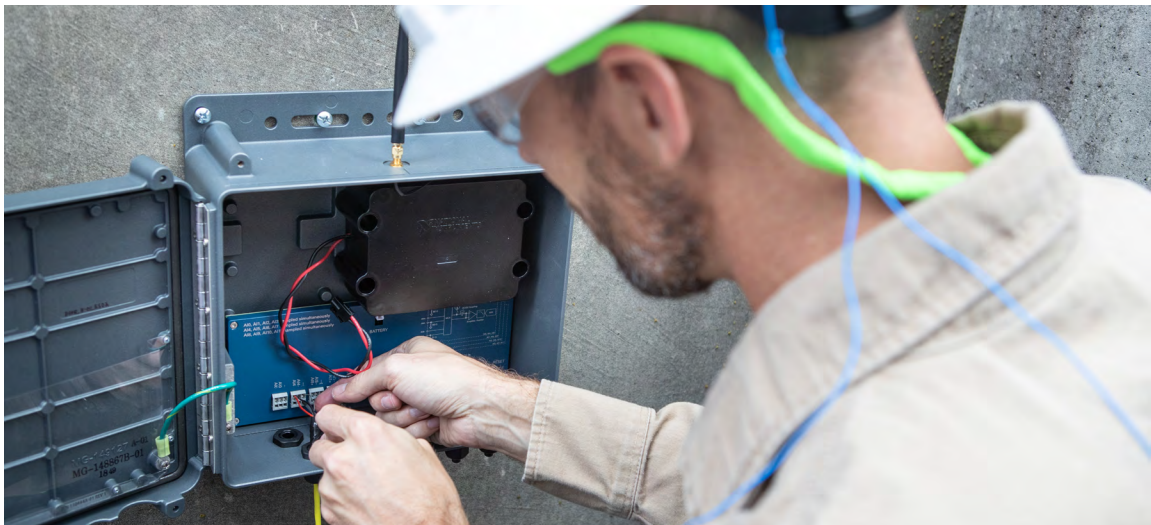
Figure 2. An engineer installs a wireless device and accelerometers to monitor three cooling towers.
